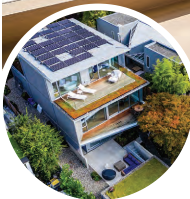
South-facing triple-glazed windows retain heat in a West Vancouver home built (by Naikoon Contracting Ltd.) for ultimate sustainability; (inset) rooftop solar panels power the family's electric vehicle, while green roofs absorb moisture.
